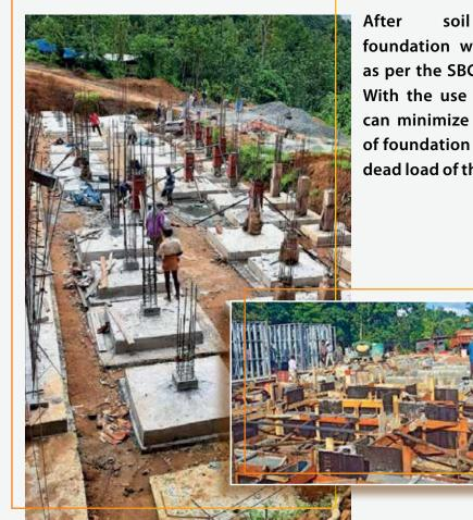
testing foundation will be done as per the SBC of the soil. With the use of LGSF we can minimize the costing of foundation due to light dead load of the structure.
